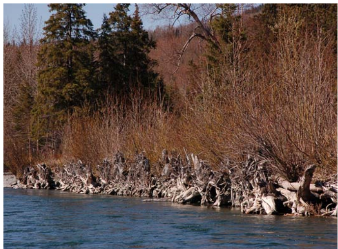
Figure 8.2 | These root wads were installed on the Kenai River in Alaska to prevent erosion. The result is a structure that looks overly symmetrical and obviously man-made, detracting from the natural scenery.
