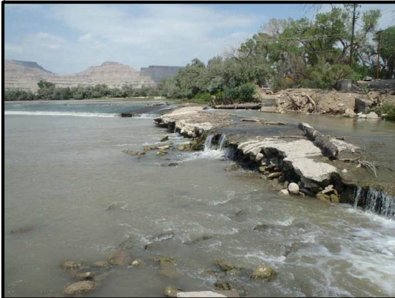
Waterwheel Raceway looking North.
