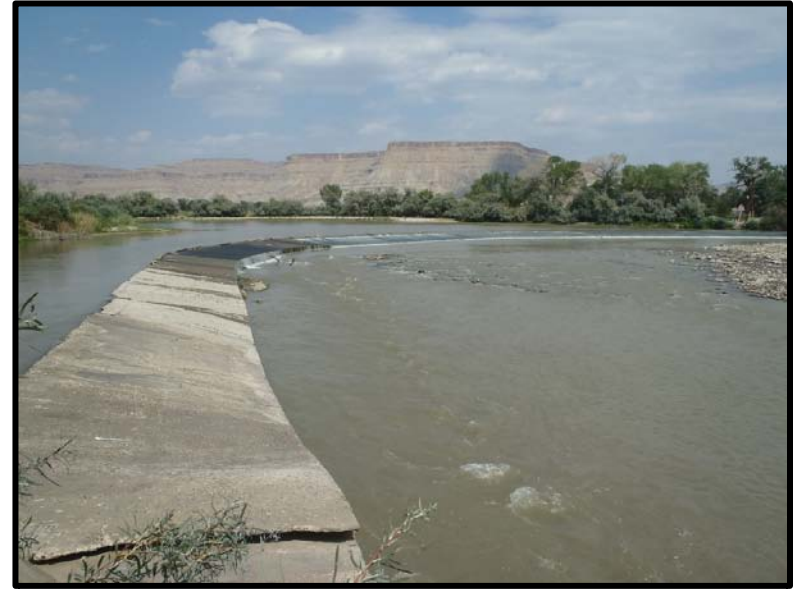
Diversion Dam looking Northeast.
