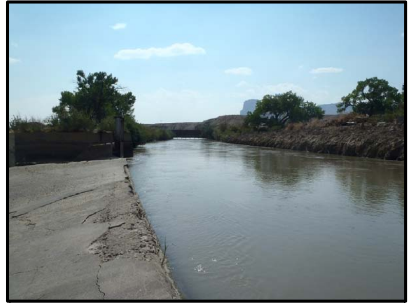
Raceway looking Downstream on West Side of Diversion.
