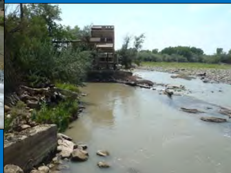
East End of Diversion Damage to Waterwheel Raceway (looking d/s)
