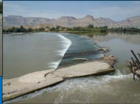
East End of Diversion
