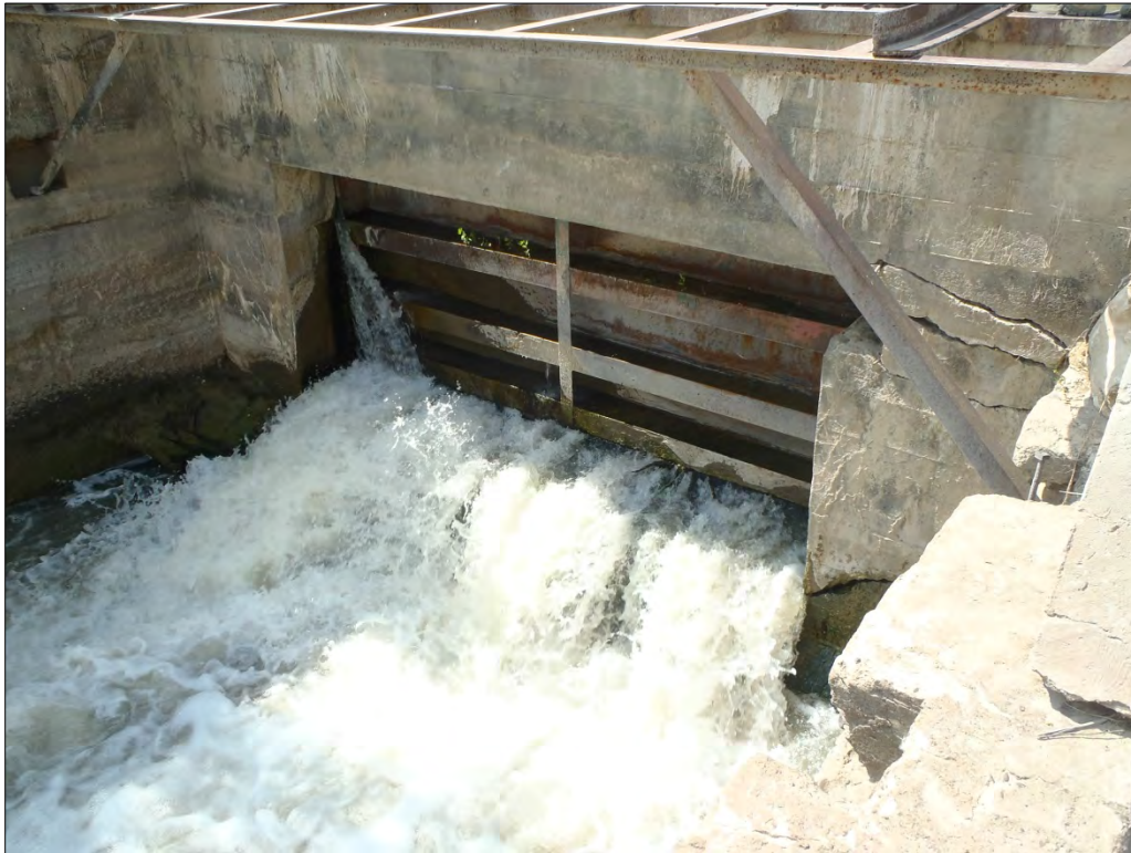
Picture 1-8. West Side Sluice Gate
