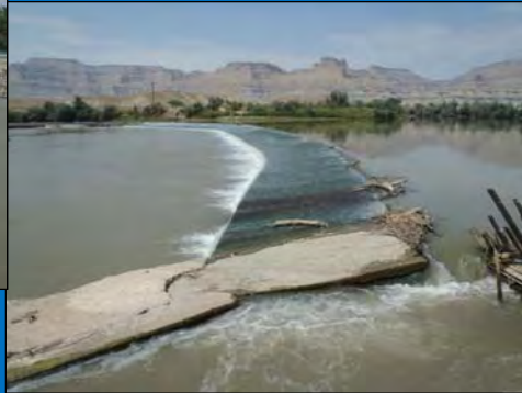
East End of Diversion
