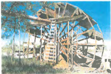
Steel Water Wheel Designed by U. of Arizona
