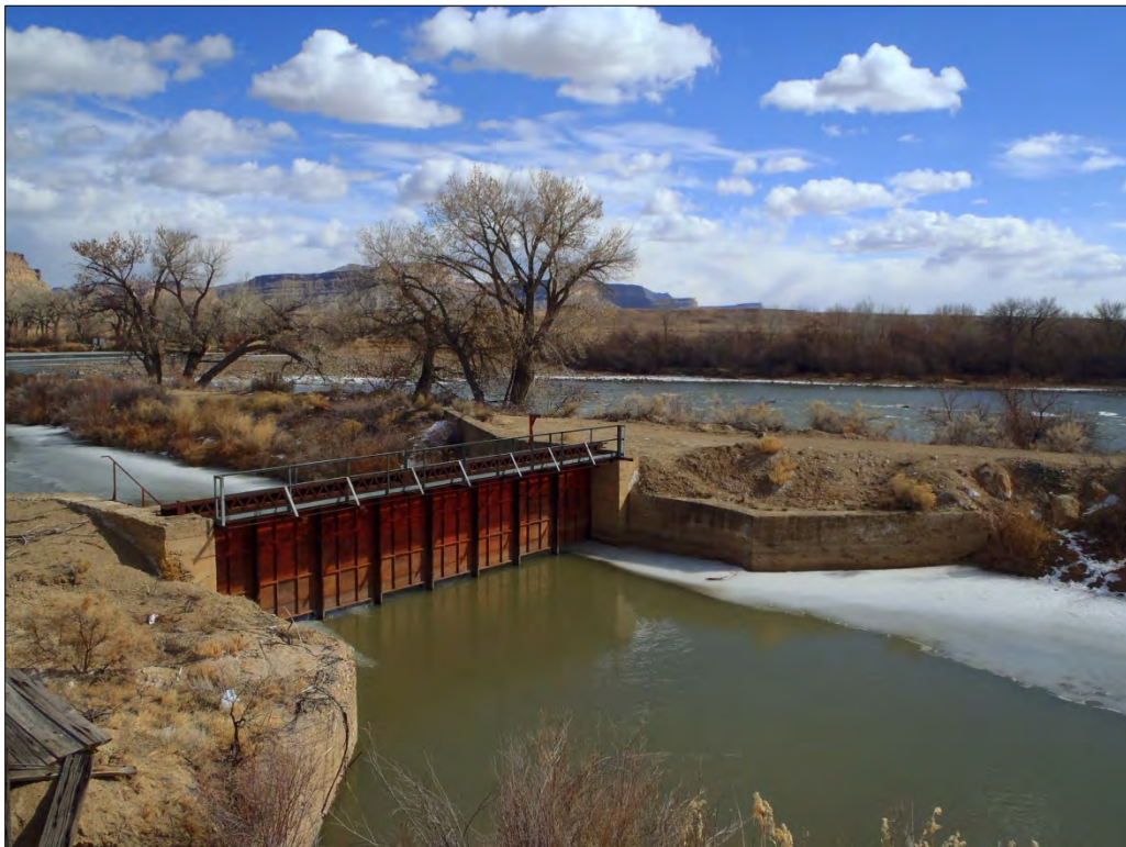
Picture 1-7. West Side Raceway Headgate Structure
