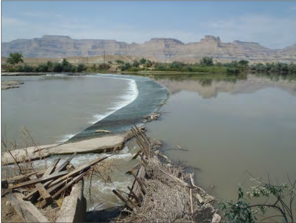
Picture 1-1. East End of Diversion
