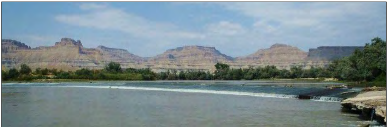
Picture 2-2. Looking North Northwest across Diversion Structure
