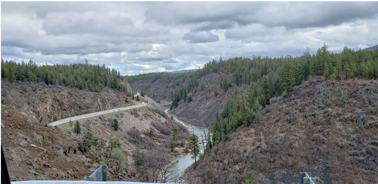
Figure 2-4: View of J.C. Boyle Bypass Reach, Klamath River Canyon and Power Canal
