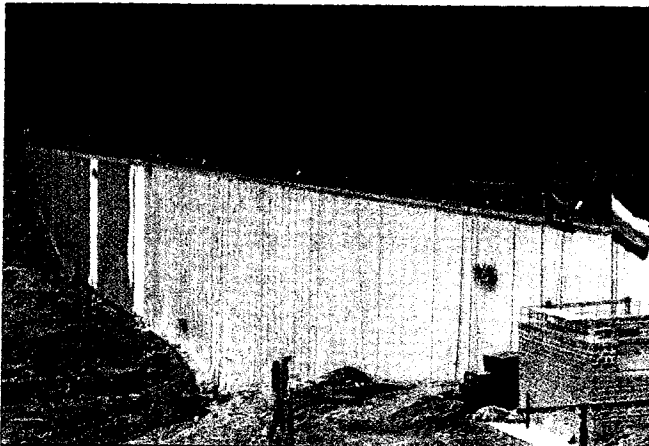
BELI ISKAR DAM - BULGARIA - 2002 Rehabilitation of a gravity dam. 14,000sq. ft. exposed PVC geomembrane installed on a steep rock masonry facing.
