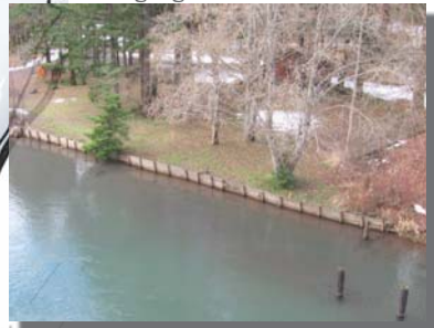
6 Existing wooden bulkhead (to be removed).
